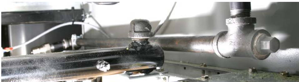
Figure 7: The T with a clean-out plug and the rear-facing discharge pipe are shown in the cabinet.
