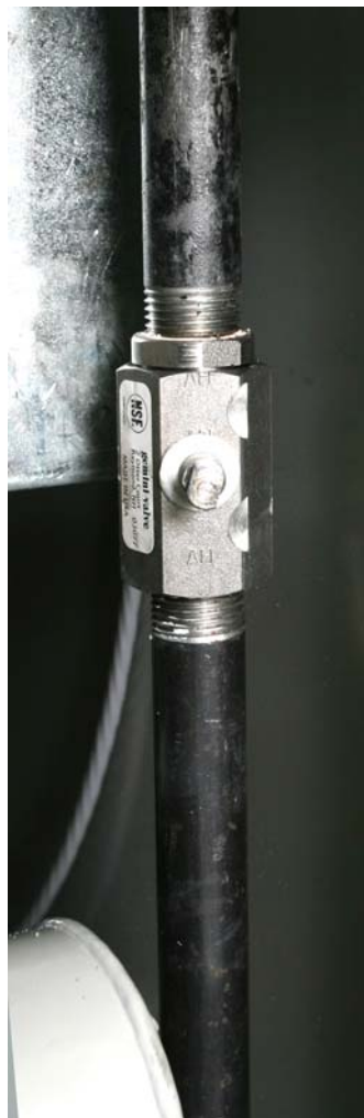
Figure 4: The valve and pipe assembly is shown partially installed in the cabinet. The valve stem will be rotated toward the corner of the cabinet before the handle is replaced.
