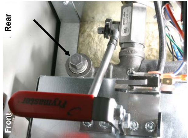
Figure 9: Looking straight up into the far right fryer cabinet, the plug in the street elbow is visible (see arrow).
