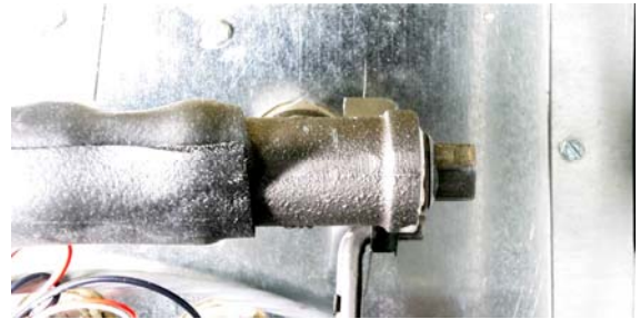
Figure 3: Remove the pipe plug from right side of the oil-return manifold.
